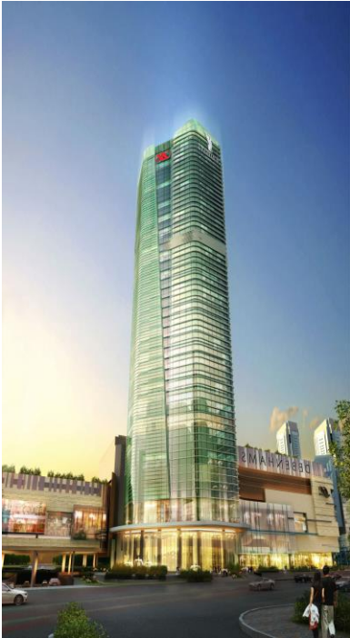
OFFICE TOWER AT THE ST. MORITZ WEST JAKARTA
